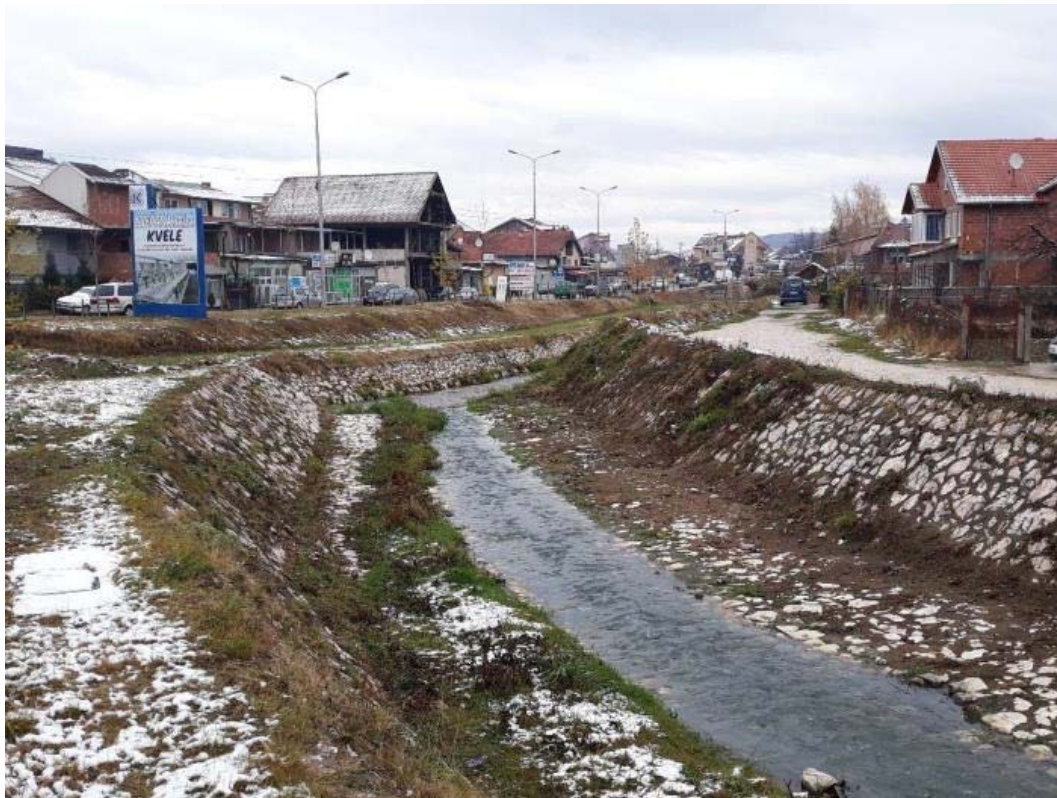
Figure 4 Trained section of Trnavica River at the confluence with Josanica
